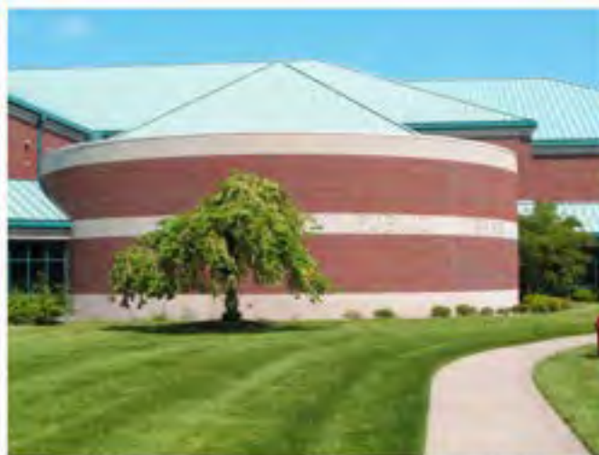
The Rochester Hills Library served over 30,000 people, and 1.5 million items circulate through the 75,000-square-foot facility each year. Photo courtesy Rochester Hills Library.
